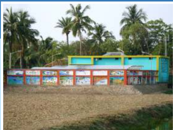
Project : Rajat Jubli Solar Power Plant Type : Off Grid
