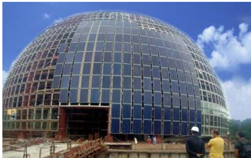
Solar Dome, 336 Kwp, Eco Park, Newtown, Kolkata
